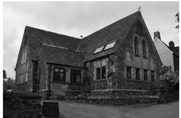
Fig. 1. Bratton Clovelly Board School. Photo © Kim Baldacchino 2013.
